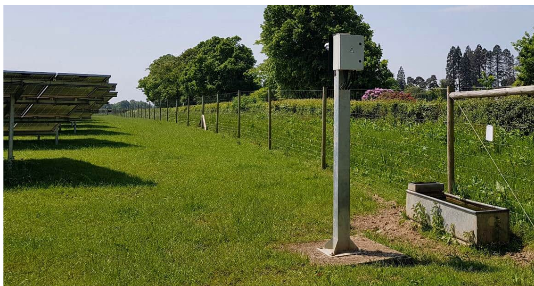
Figure 2-11: Metal CCTV pole and 'deer fence'
