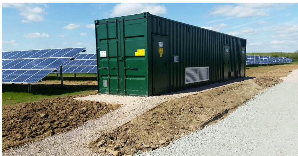
Figure 2-8: Example field substation
